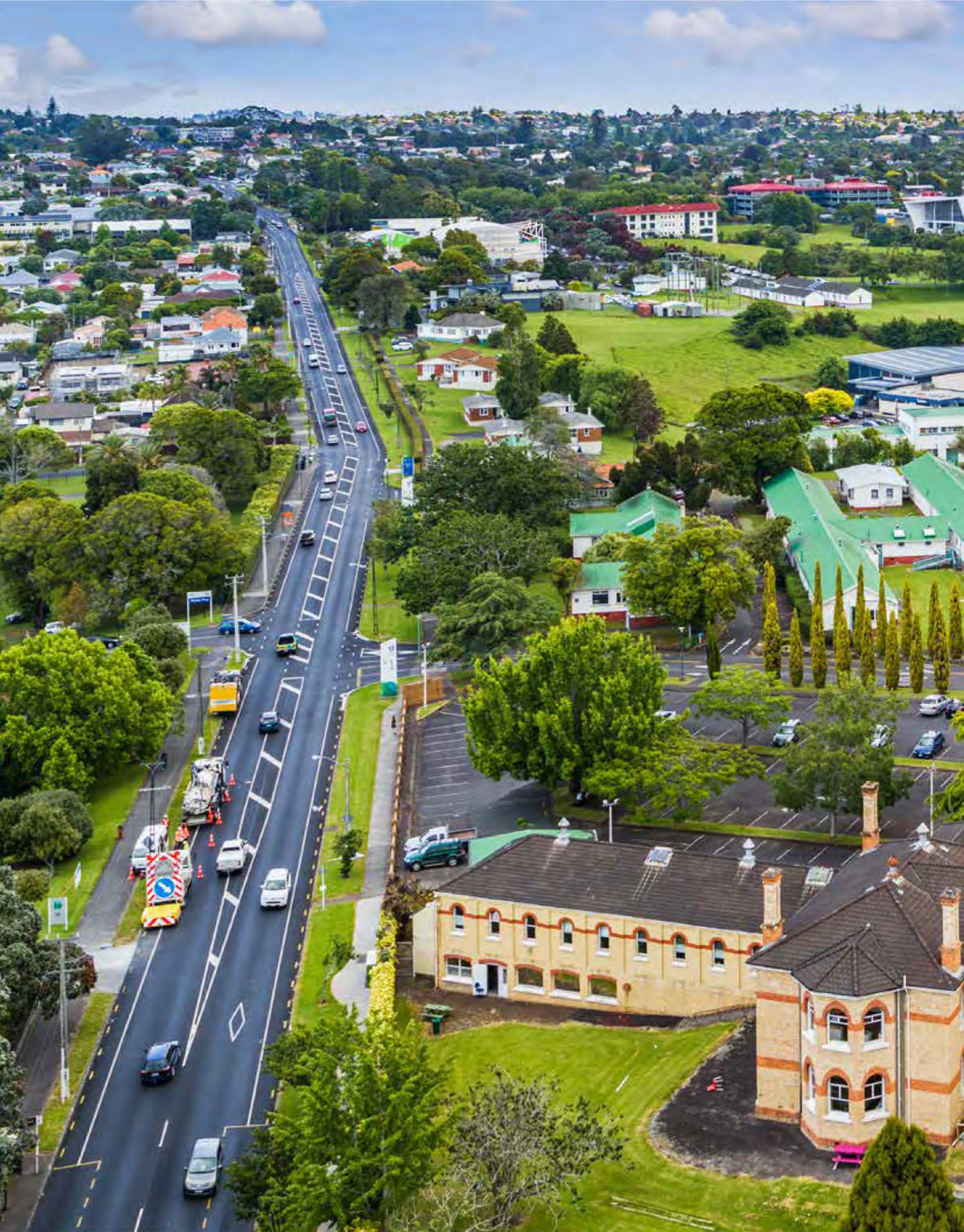
Aerial view of site looking South along Carrington Road
