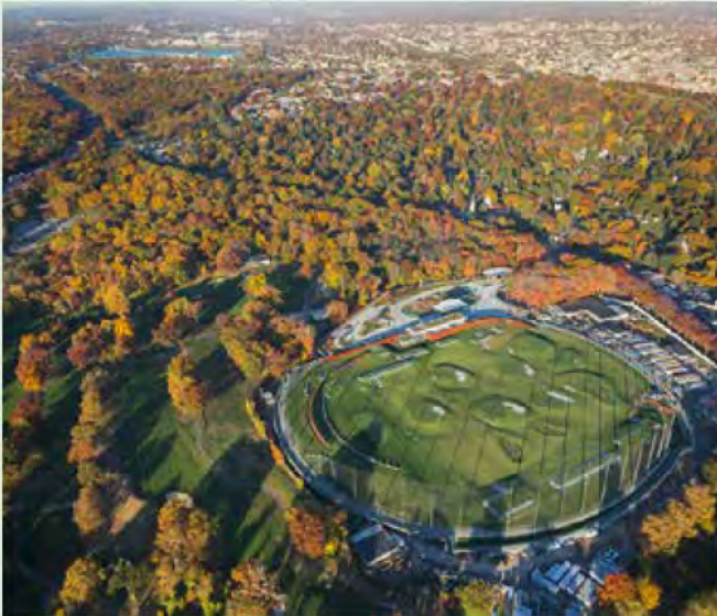
Croton Water Treatment Works – New York
